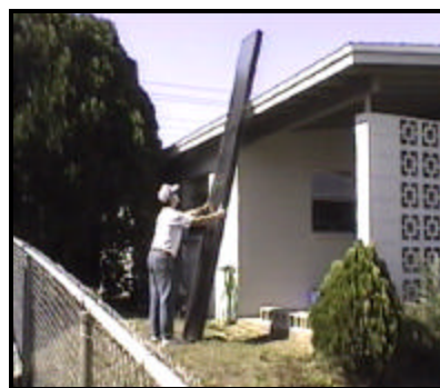
Protect Edge of Roof with a Tarp and Lean Collector Against Roof
