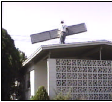
Balance the Collector in the Center and Carry to Installation Area.
